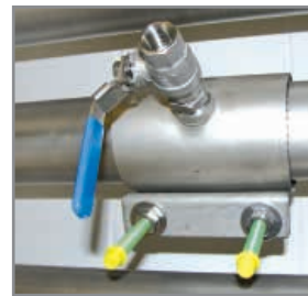
B Spot drilling collars
