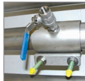
B Spot drilling collars
